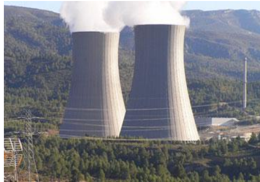
SDI Power Station, Valencia, Spain
