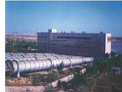
Uzbekistan Tusterrick Pumping Station Project
