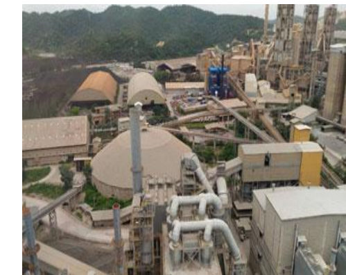
TPI PP 150MW Power Plant In Thailand
