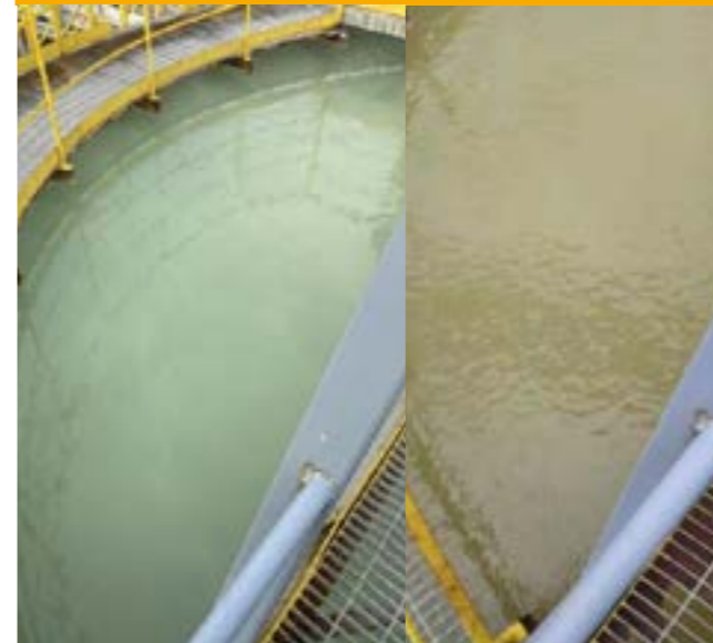
▶ Comparison of wastewater before and after treatment
