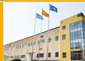
↖ Catalyst Production Plant (Tianjin)
