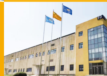
↖ Catalyst Production Plant (Tianjin)
